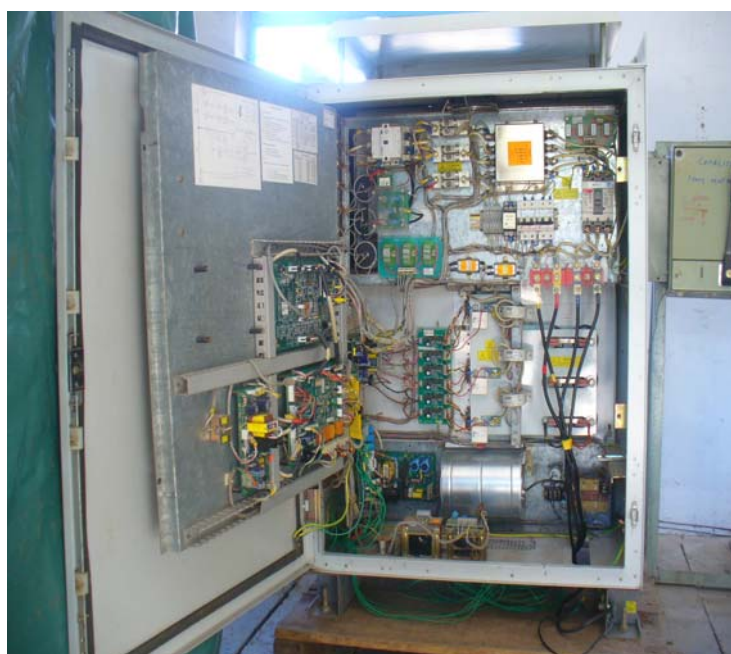
Harmonic Filter DAPC-Panel 60 (Diesel Generator at 750KVA Set)
